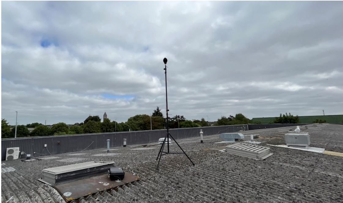
Figure B2 UT1 Installation
