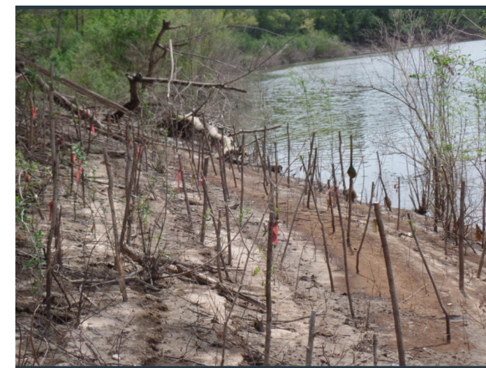
Above(Left and Right): Live willow Staking BioengineeringTechnique
