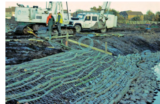
Above (Left and Right): Live Willow Mattress Bioengineering Technique
