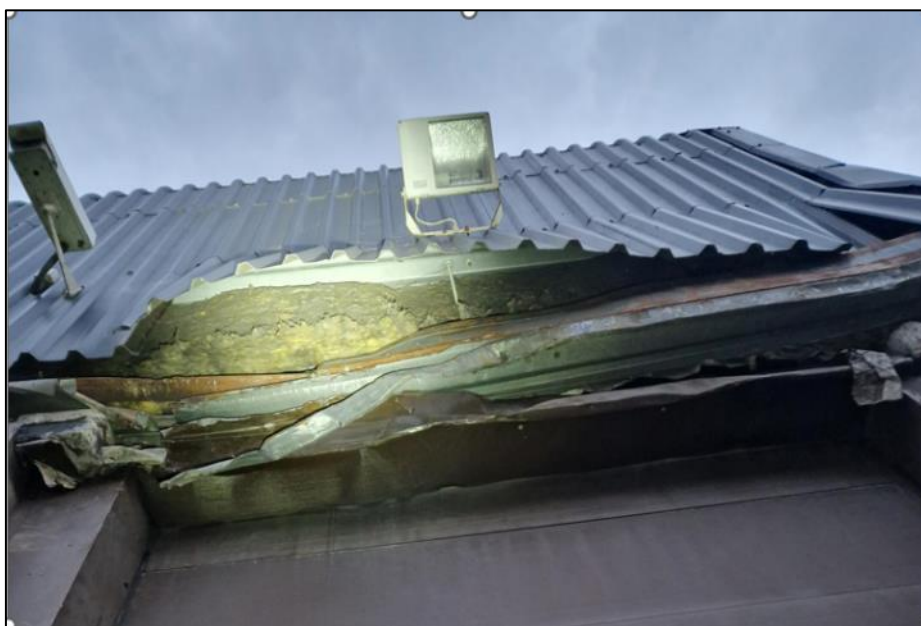
FIGURE 7. DAMAGE TO THE EXTERIOR OF THE MAIN BUILDING WHICH MAY PROVIDE ROOSTING OPPORTUNITIES FOR BATS.
