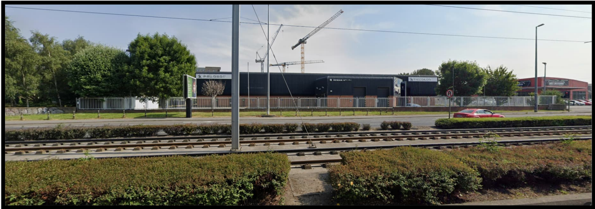
Figure 2-1: Front View of The Site From Naas Road
