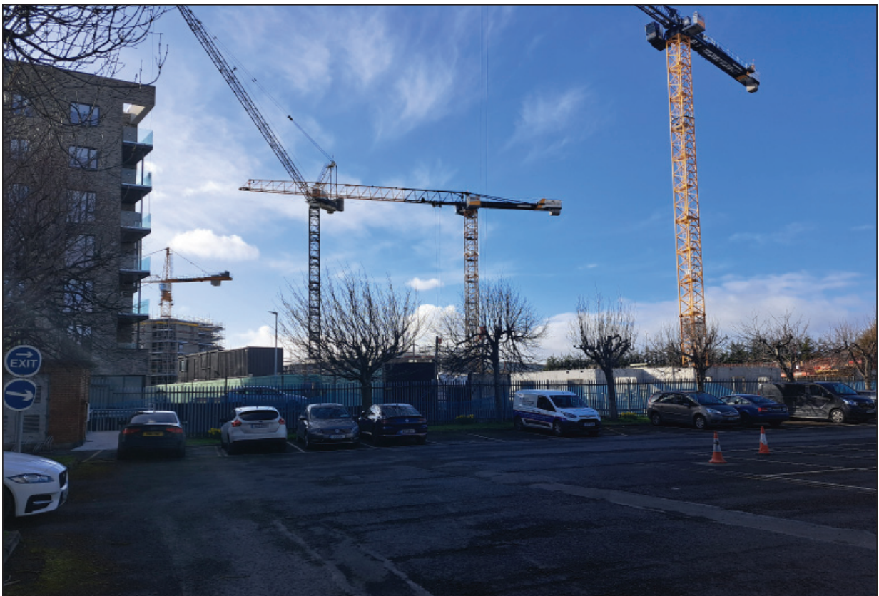
Plate 4 - View of Carriglea Industrial Site from proposed development site (towards Drimnagh Castle CH005 and CH010-CH014), facing southeast
